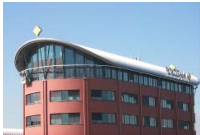
Curved installation for window cleaning equipment
