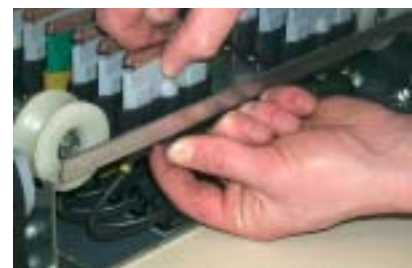
Replacing the carbon brushes.
